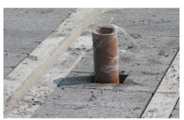
Services must not be attached to the beams or blocks in such a way as to impact on their strength or durability.
