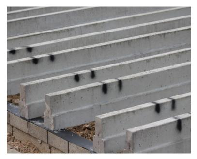
On ground floors a continuous damp-proof course must be laid along the top of the support wall, before the beams are lifted into position. To ensure a clean bearing on the support wall and to avoid damage to the DPC, the underside of the beams should be cleaned of dirt or debris before they are placed in position.
